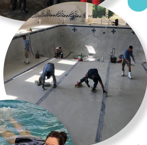
Pool Resurfacing Project, Aug-Sept 2022
